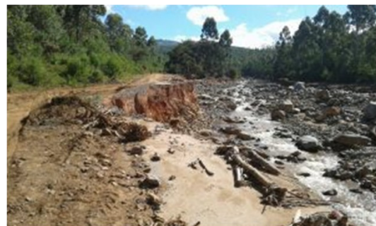
The cyclone and aftermath washed out roads, like this one on the way to Charleswood.
